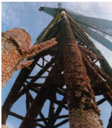
Figure 3. Examples of damages to structural integrity: biofouling on an offshore jacket foundation (left); schematic representation of different stages in marine biofouling process (right) (Davies & Williamson, 1995)
